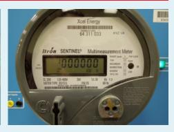
This is a standard meter that determines how many kWh your solar system is producing each month. Monthly statements are sent to the owner of the PV system. Production Meters are installed on systems greater than 40 kW AC.
